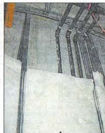
Photo shows wall insulation being placed over uninsulated hot and cold water pipes. — HANDOUT
